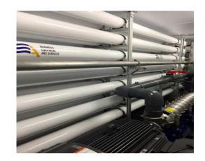
ARKQUA® systems are built in a standard 40' ISO container, R19 thermal and acoustic insulation protects equipment from temperature fluctuations and prevent noise which can disturb the environment. Systems are engineered for fast deployment integrating the most energy efficient components.
