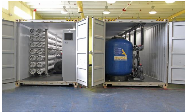
CONTAINERIZED SEAWATER DESALINATION SYSTEM – 1500M3D/400.000 GPD
